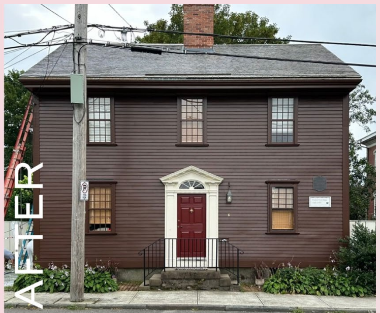
The BEFORE and AFTER photographs of 6 Elm Street show clapboard replacement in process and then the finished exterior with a new coat of paint.
